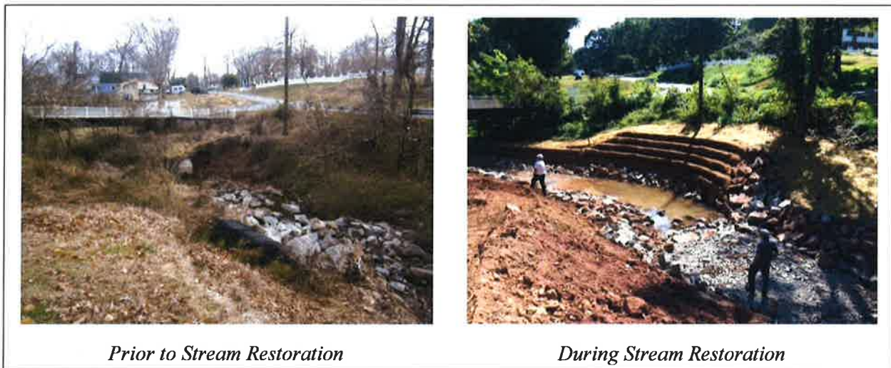
Figure 2B – Oak Street Stream Restoration Project
