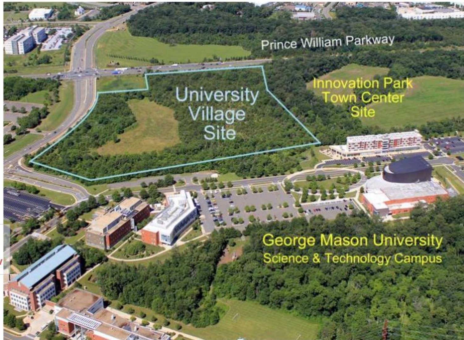
Both a "University Village at Innovation" and a "Town Center at Innovation Park," with a total of more than 2,600 student housing units, apartments and townhomes, has been approved near George Mason University's Manassas campus.
