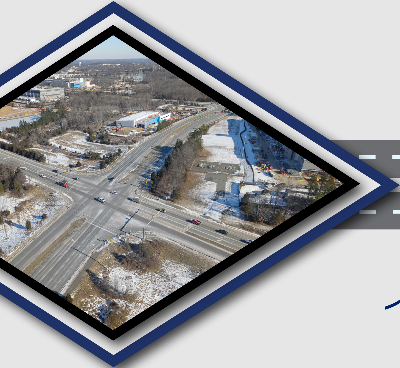
ROUTE 234 AND SUDLEY MANOR DRIVE INTERCHANGE
