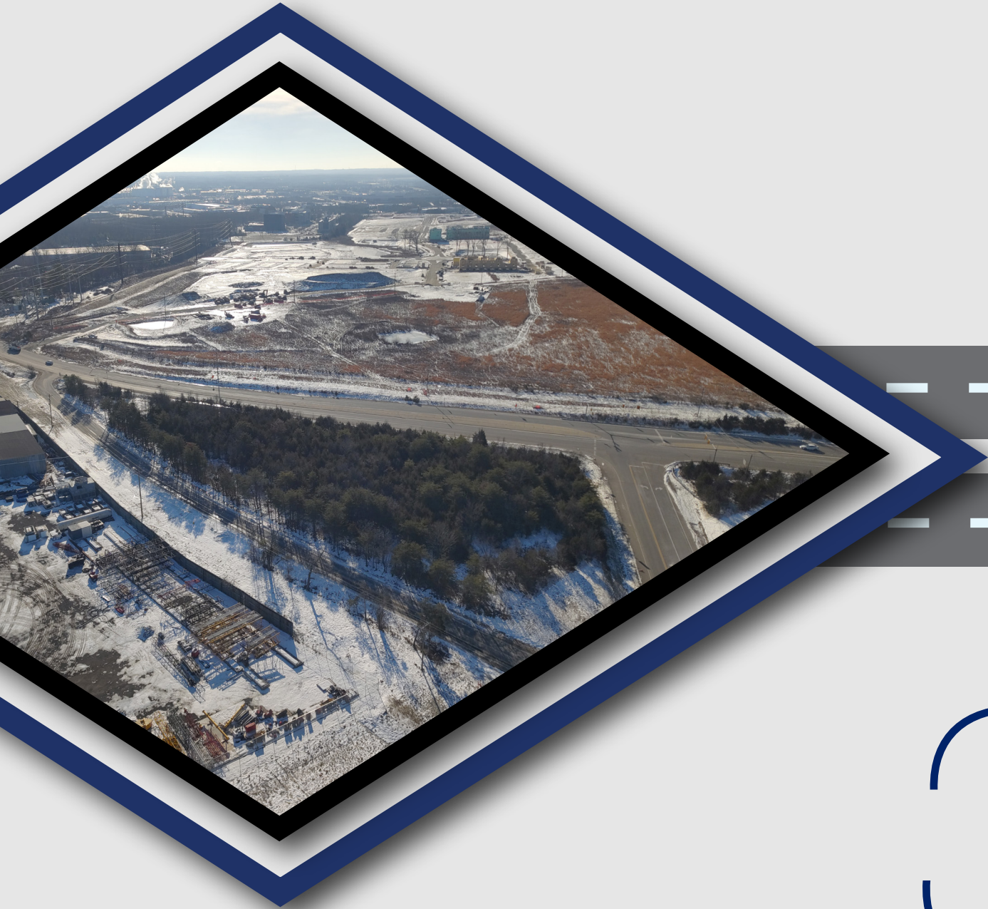
ROUTE 234 AND SUDLEY MANOR DRIVE INTERCHANGE
