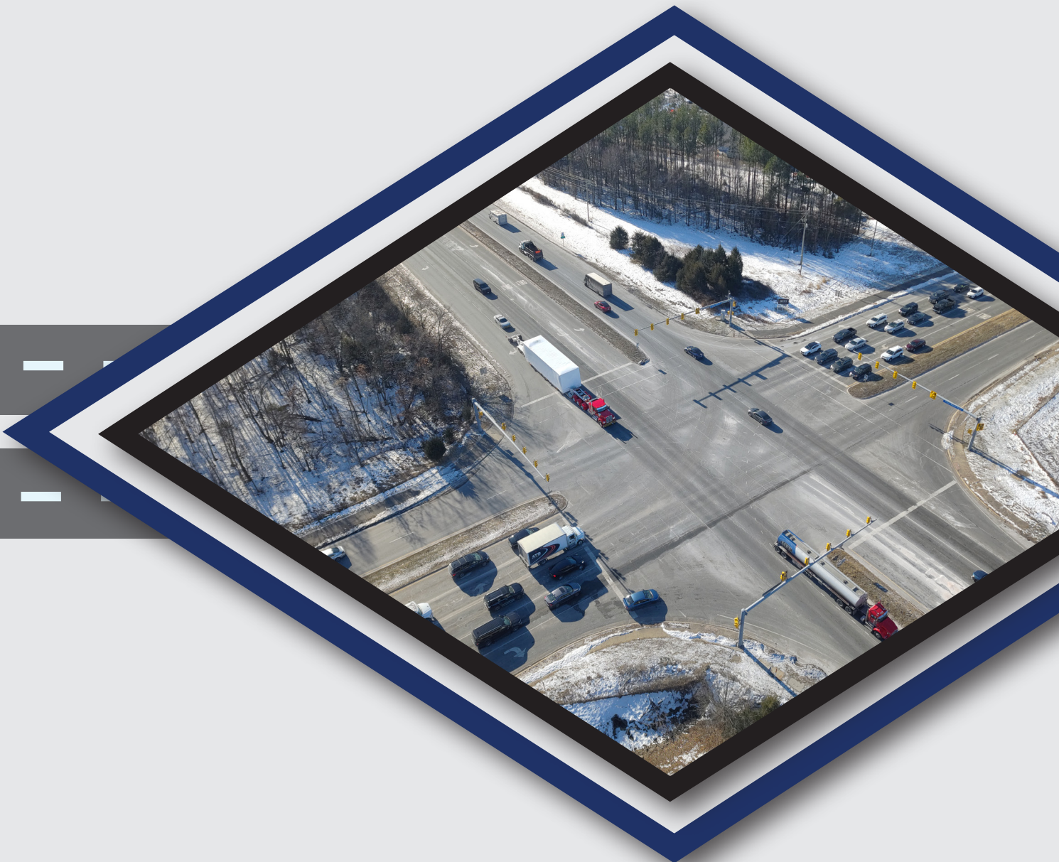
ROUTE 234 AND SUDLEY MANOR DRIVE INTERCHANGE
