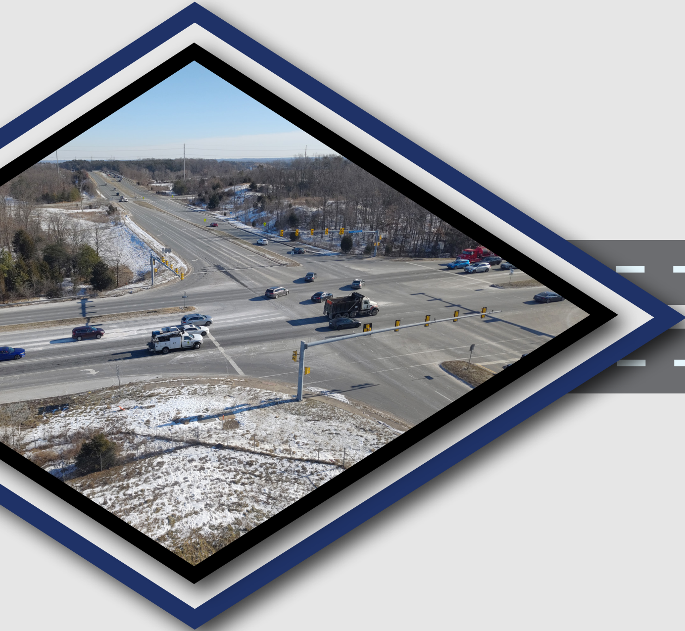
ROUTE 234 AND SUDLEY MANOR DRIVE INTERCHANGE
