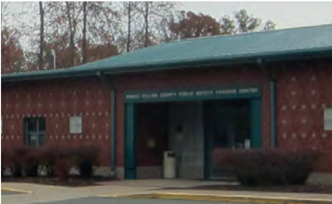
figure 3-3 | Joint Training Building
