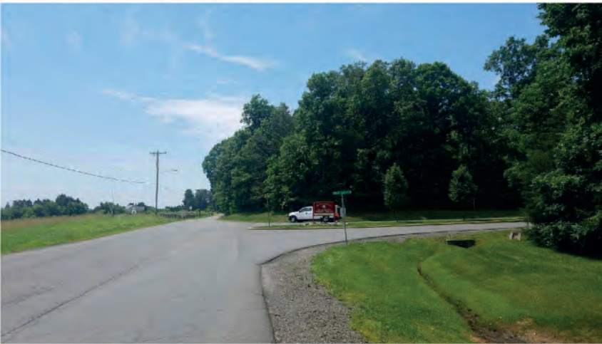
FIGURE 4. Southbound View of Access
