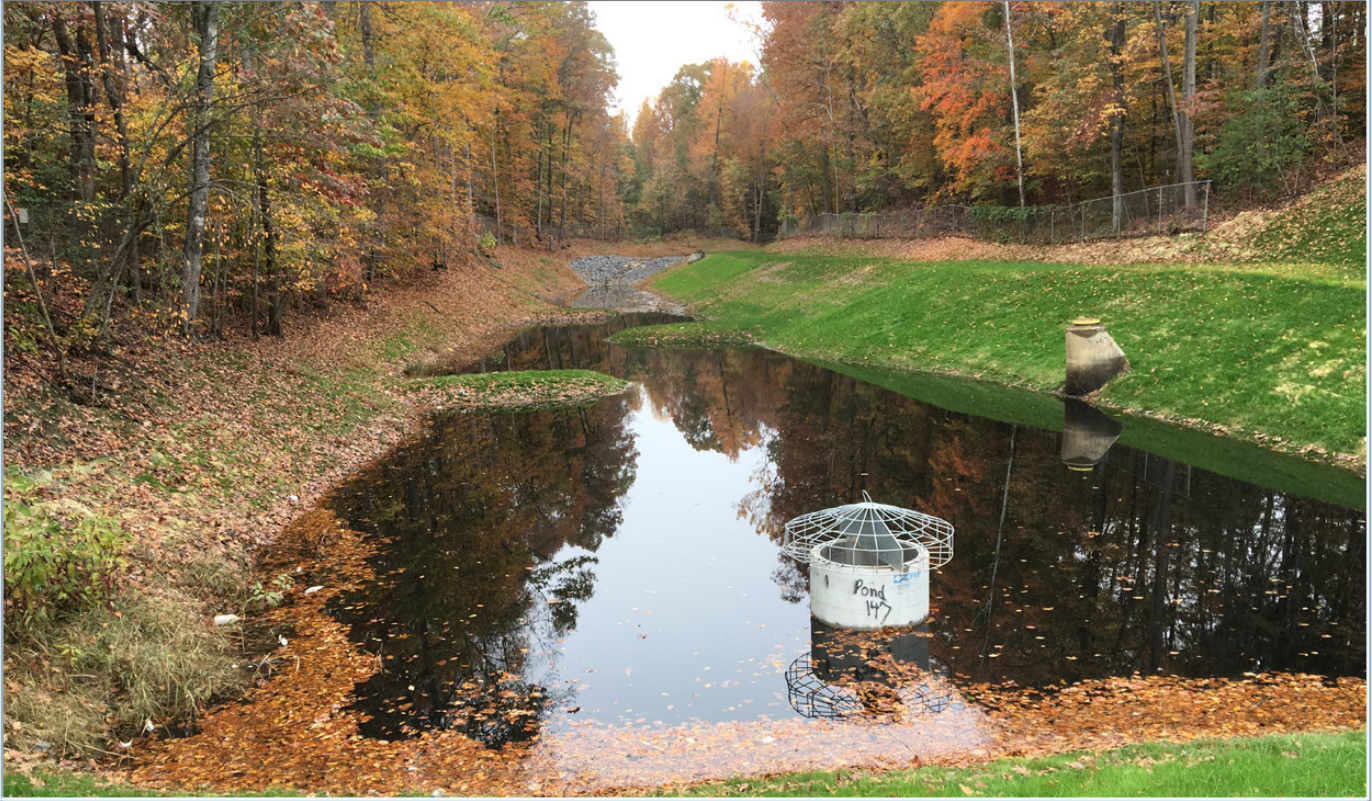
Powells Creek Watershed Water Quality Retrofit
