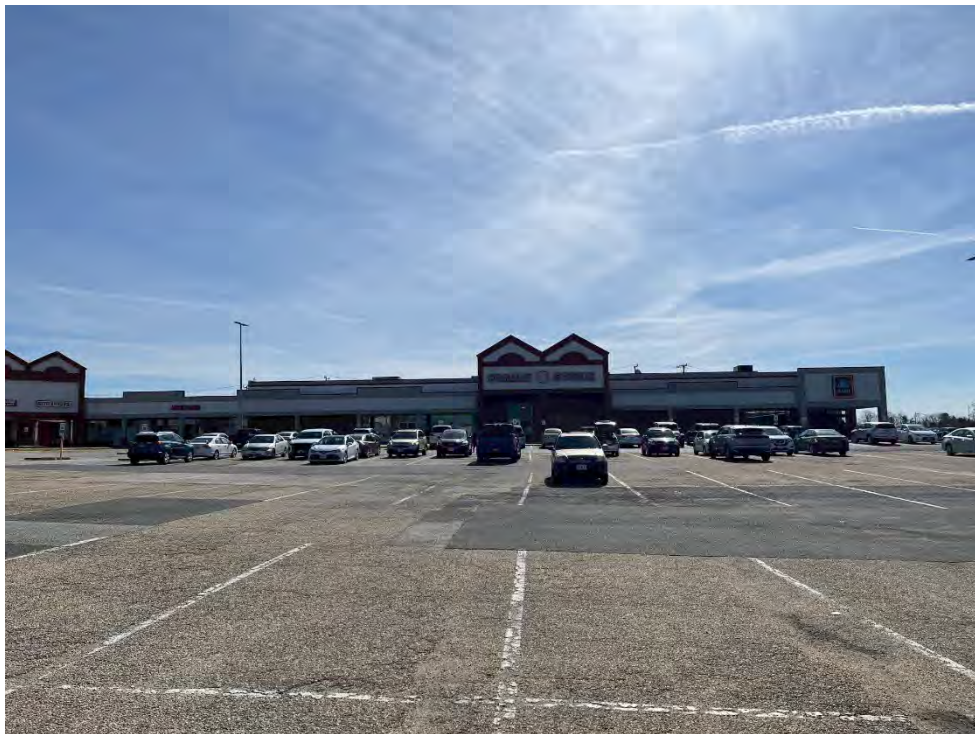
Photograph # 28 - Gordon Plaza South Building Exterior (3/1/2024)
