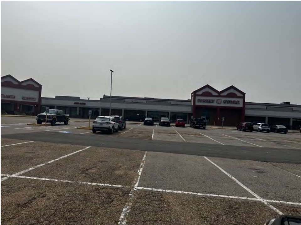
Photograph #2 - View of onsite buildings from west (7/13/2023)
