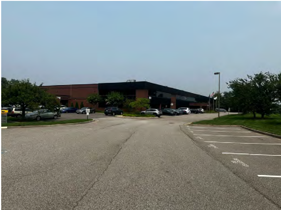
Photograph #18 – Office building located to the northwest, adjacent to property (7/13/2023)
