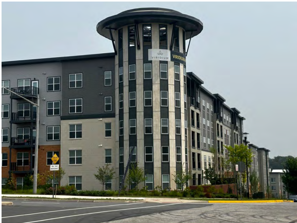
Photograph # 16 - Residential development on north adjacent property (7/13/2023)
