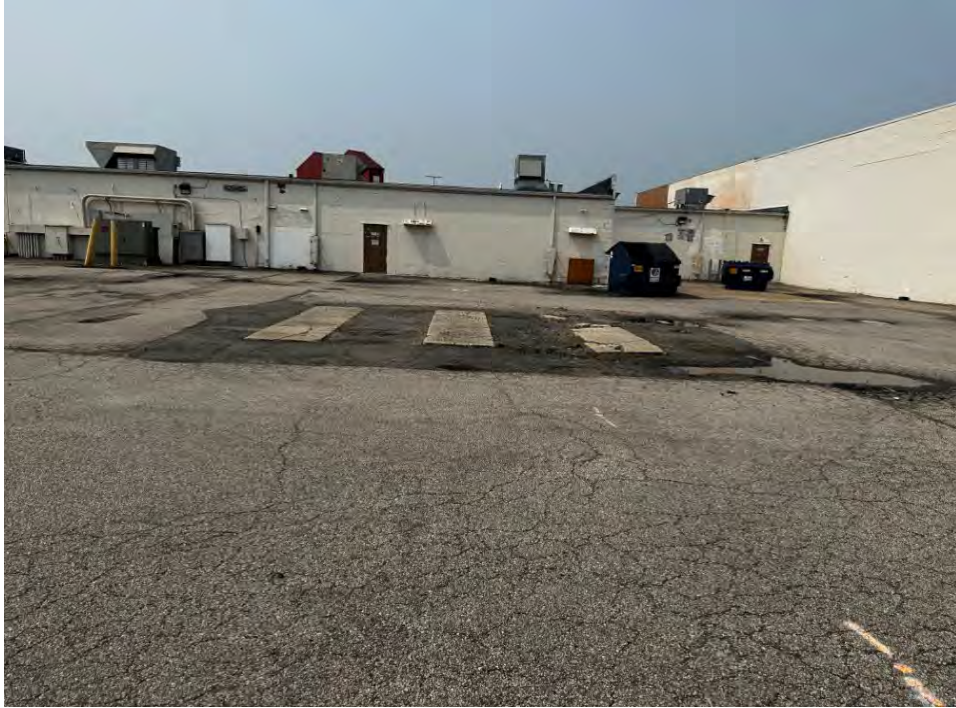
Photograph # 11 - Rear/north side of onsite buildings (7/13/2023)
