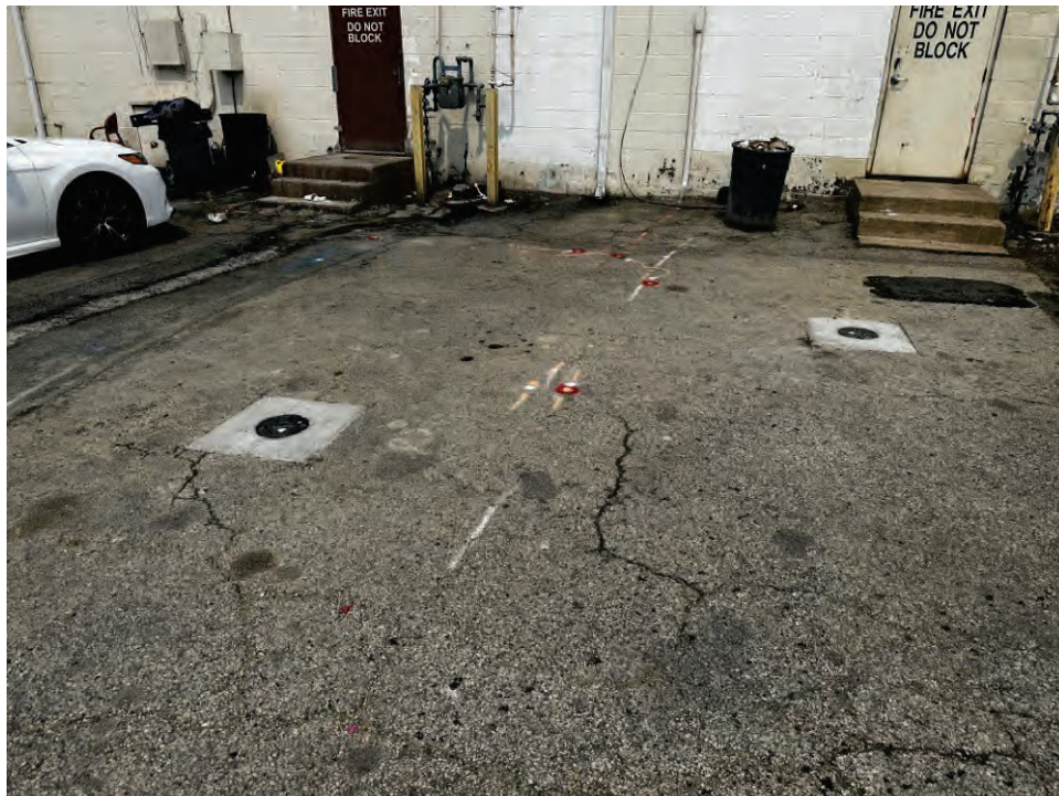
Photograph # 10 - Groundwater monitoring wells observed on north side of onsite buildings (7/13/2023)
