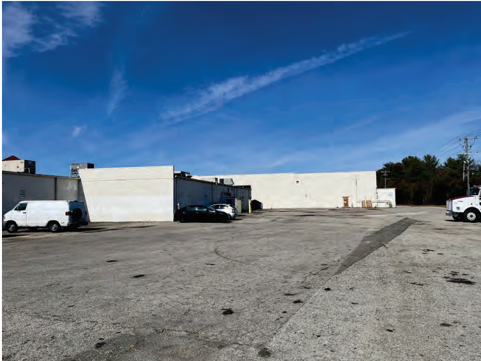
Photograph # 30 - Rear exterior of Gordon Plaza Main Building (3/1/2024)
