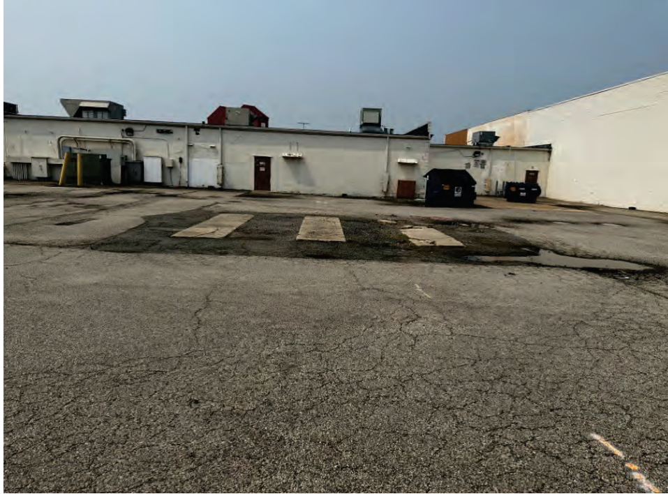
Photograph # 11 - Rear/north side of onsite buildings (7/13/2023)
