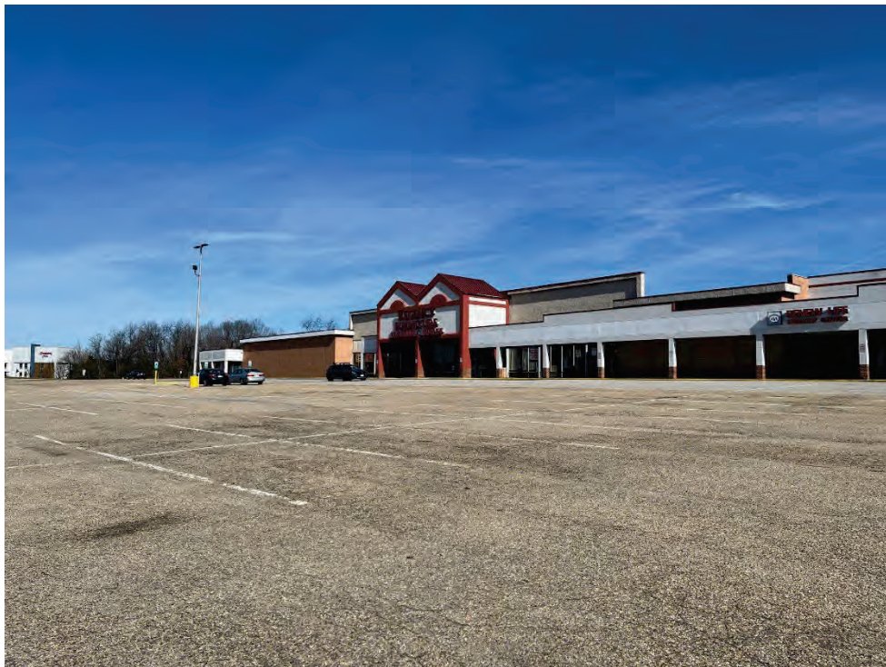
Photograph # 26 – Gordon Plaza Main Building exterior; west side (3/1/2024)
