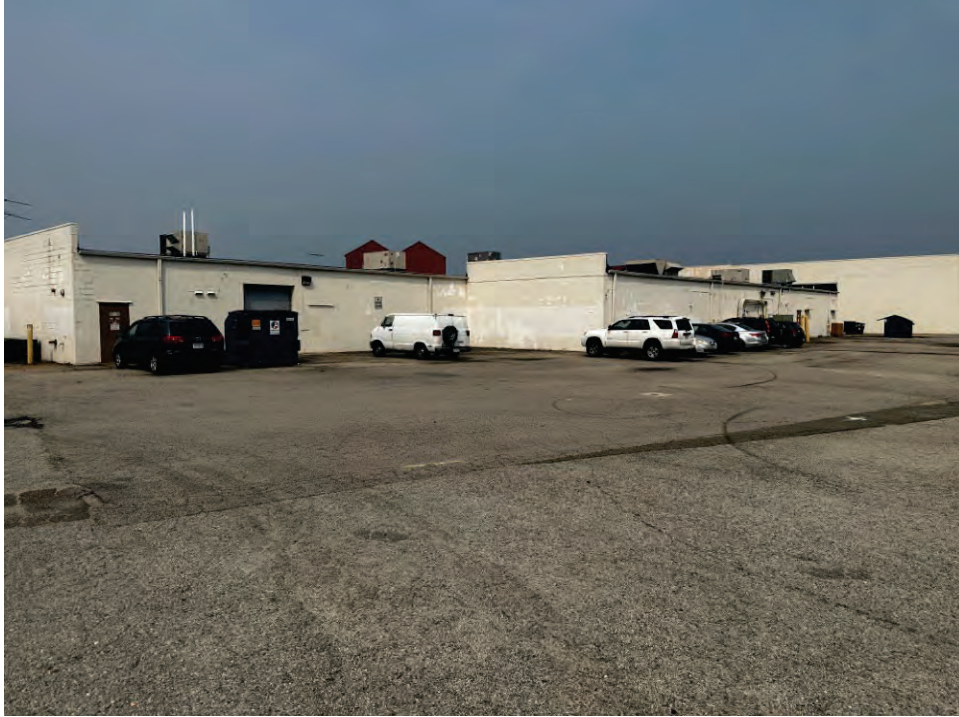
Photograph #3 - View of rear (north) side of on-site buildings (7/13/2023)
