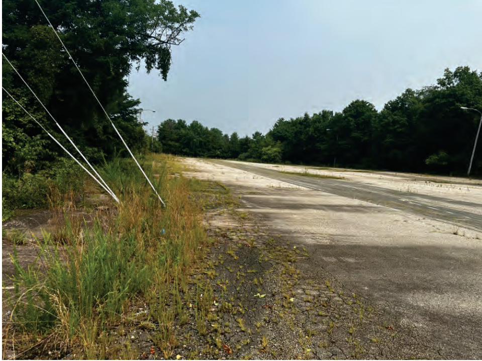
Photograph # 7 - Asphalt paved area located in central portion of property. (7/13/2023)
