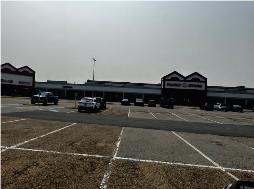
Photograph #2 - View of onsite buildings from west (7/13/2023)
