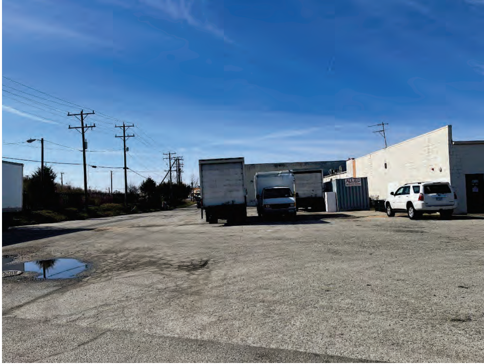
Photograph # 29 – Rear exterior of Gordon Plaza South Building (3/1/2024)
