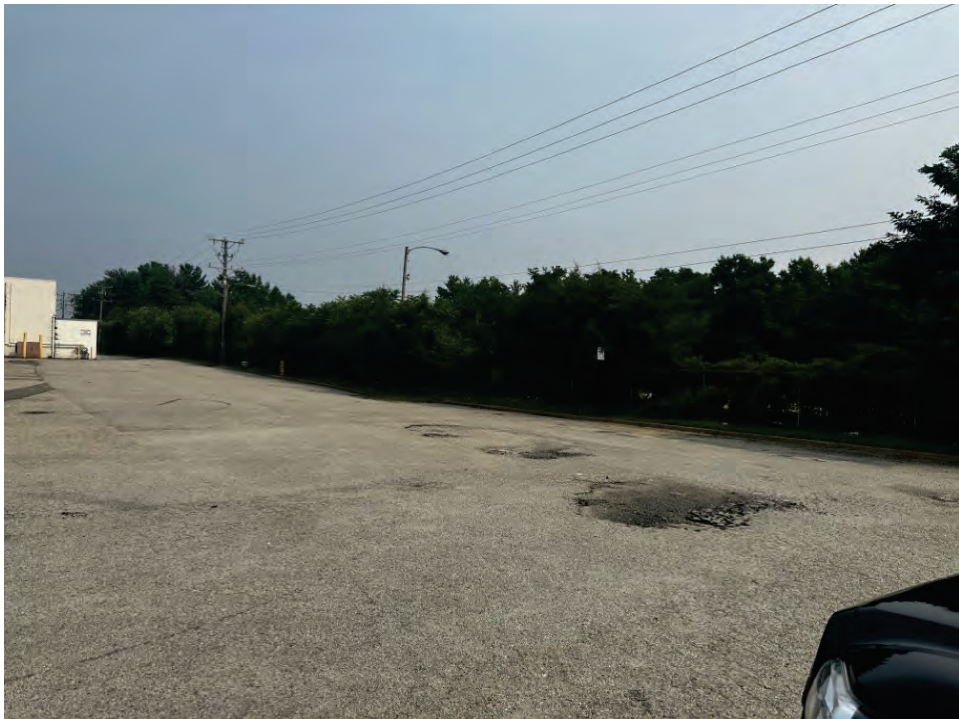
Photograph #4 - Asphalt parking area in central area of site, immediately north of commercial buildings (7/13/2023)
