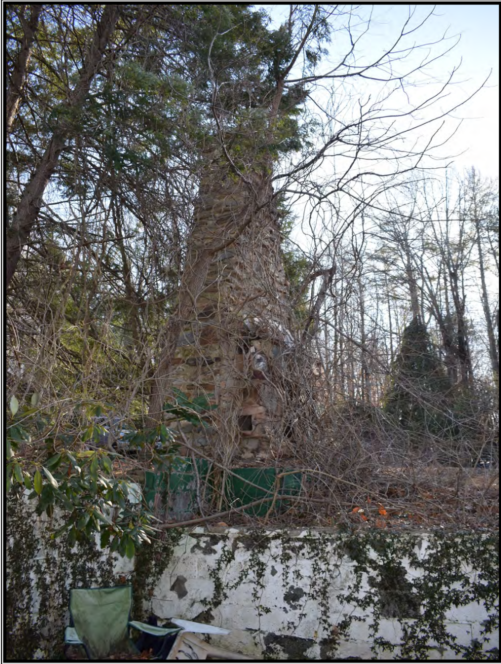
Plate 33. View of the stone chimney and foundation, looking southwest.
