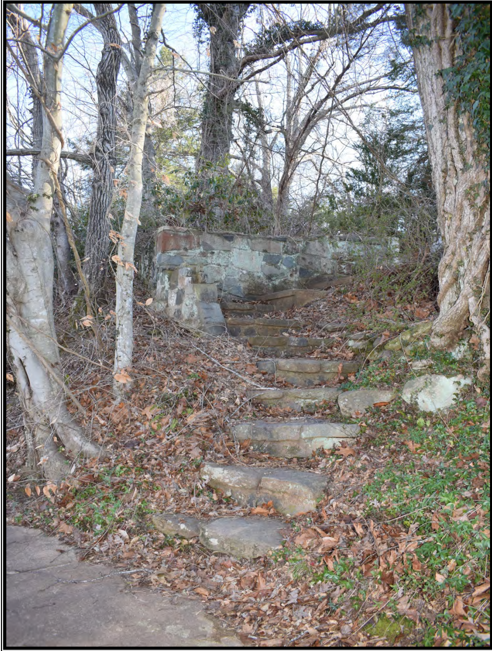
Plate 41. View of the landing, looking southeast.
