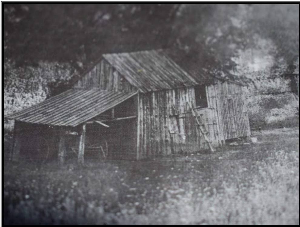
Plate 46. Detail view of barn/stable (photo in landowner's collection).
