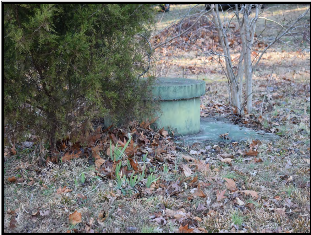
Plate 36. View of the well and iris, looking east.
