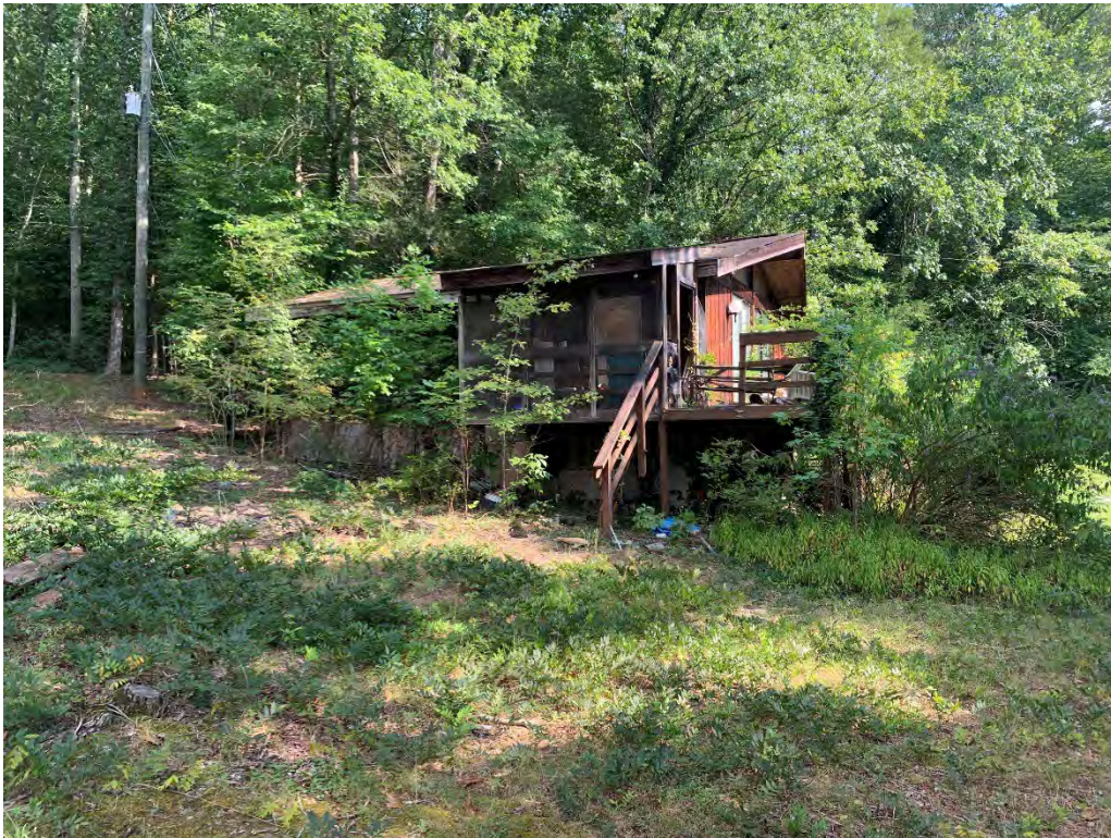
Photograph 18: Circa 1978 Dwelling Overlooking Lawn to South. View east (MN 8/29/2024).
