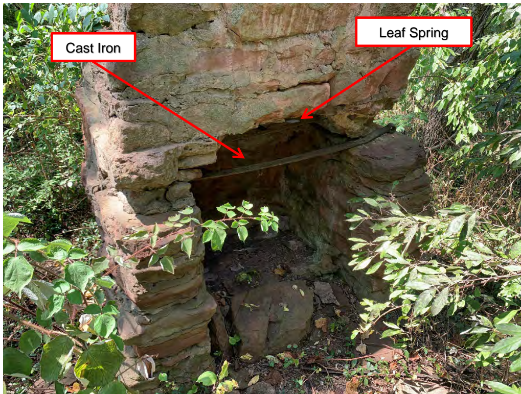
Photograph 10: Chimney Interior with Cast Iron Furnishings. View south (MN 8/29/2024).
