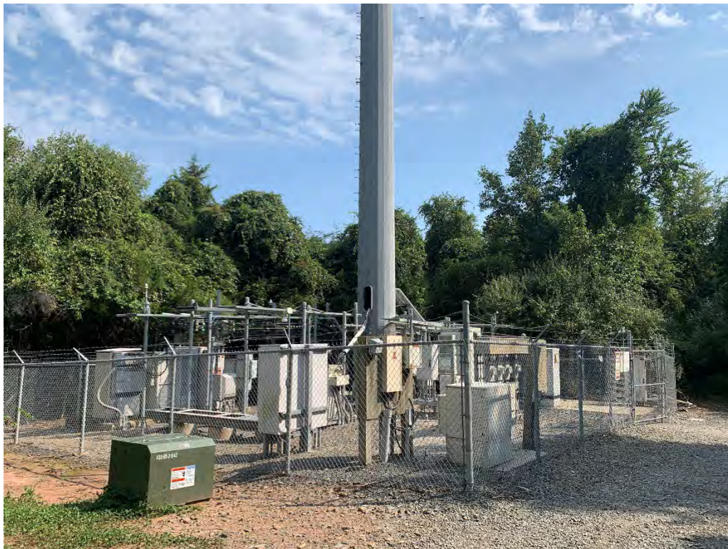
Photograph 6: Cell Tower Within the APE. View south (MN 8/29/2024).
