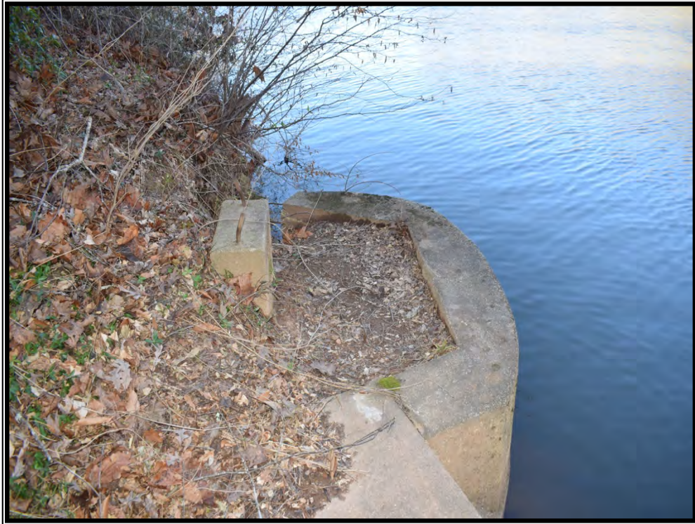
Plate 39. View of the landing, looking west.
