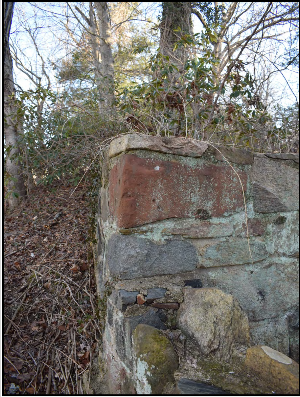
Plate 42. View of retaining wall at the landing, looking east.
