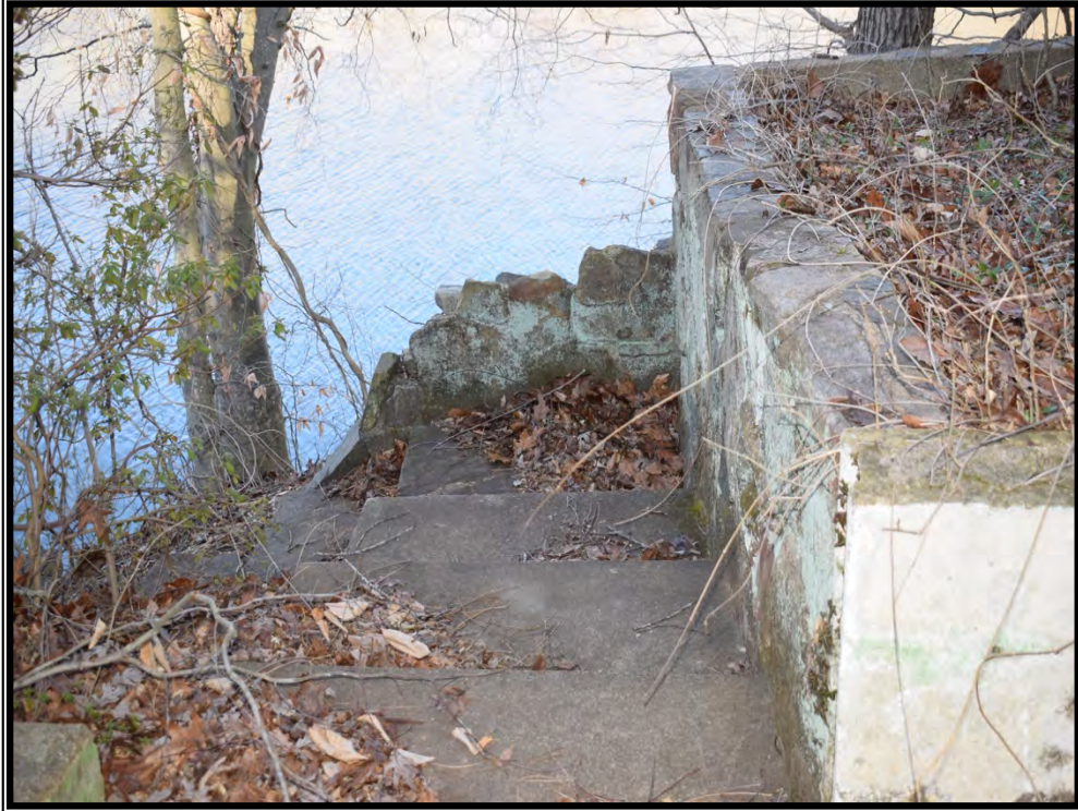
Plate 37. View of the landing, looking north.
