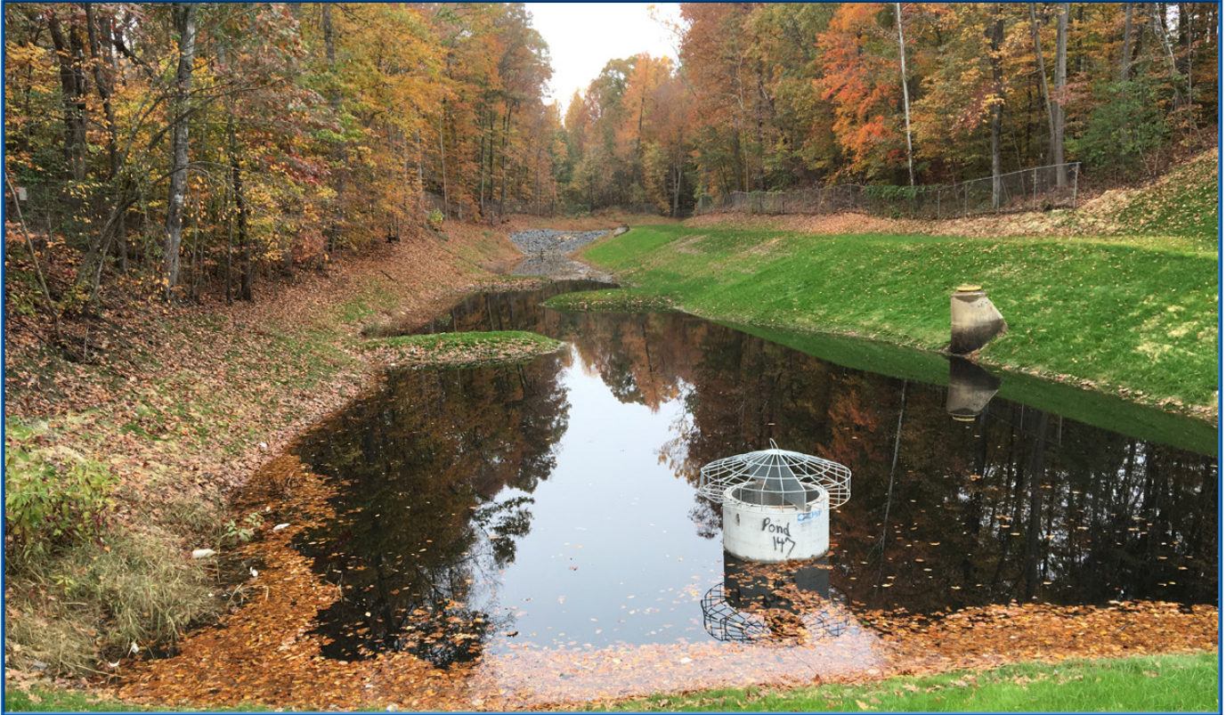
Powells Creek Watershed Water Quality Retrofit
