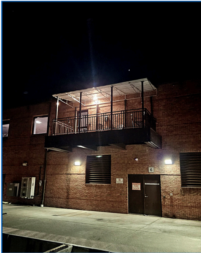
Owens Building Balcony Repair
