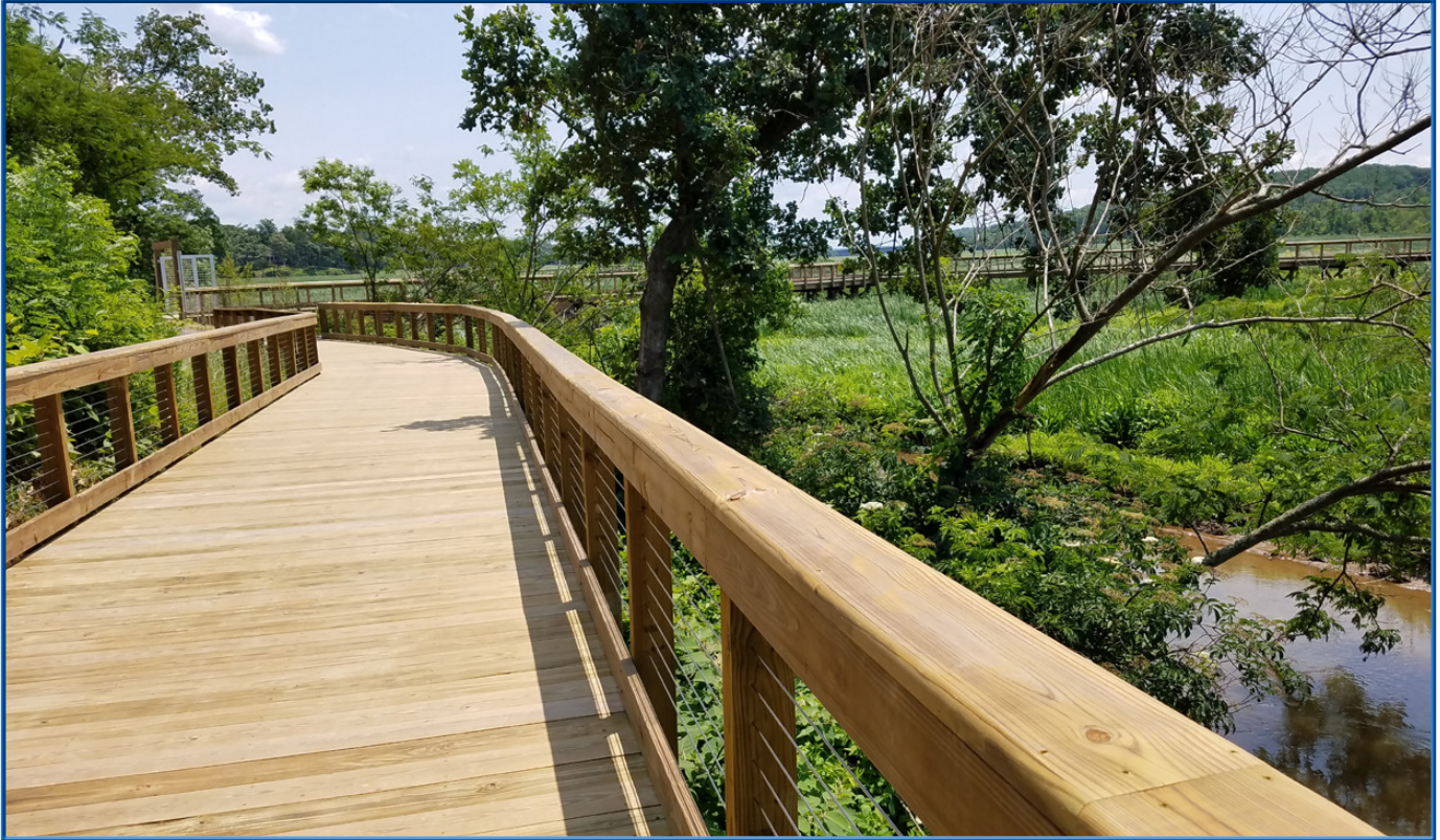
Neabsco Creek Boardwalk
