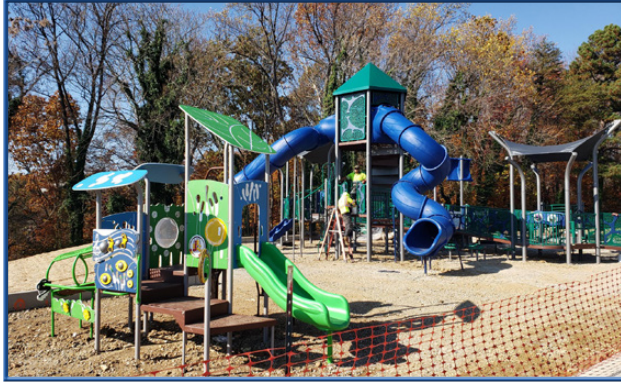
Birchdale Park Playground - Shelter Replacement
