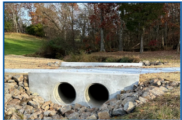
Prince William Golf Course Culvert Repair
