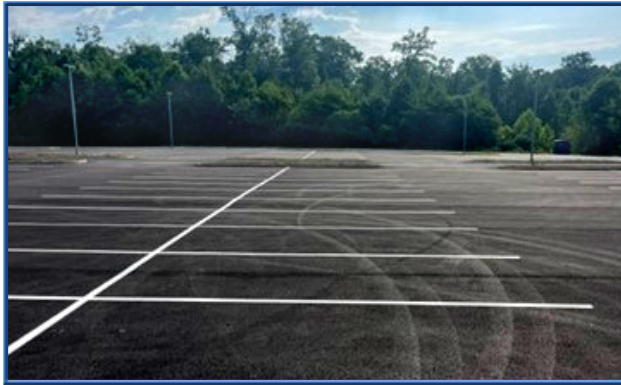
Catharpin Park Parking Lot Paving
