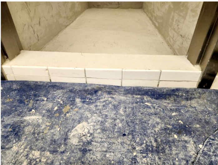
Shower floors before
