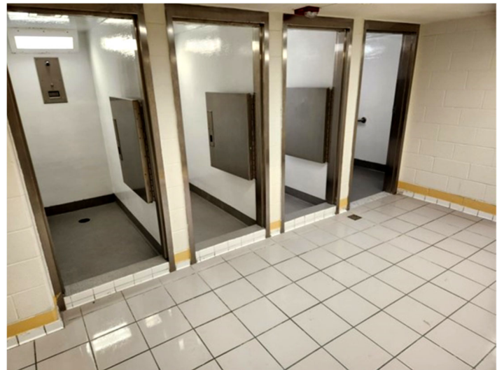
Shower floors after
