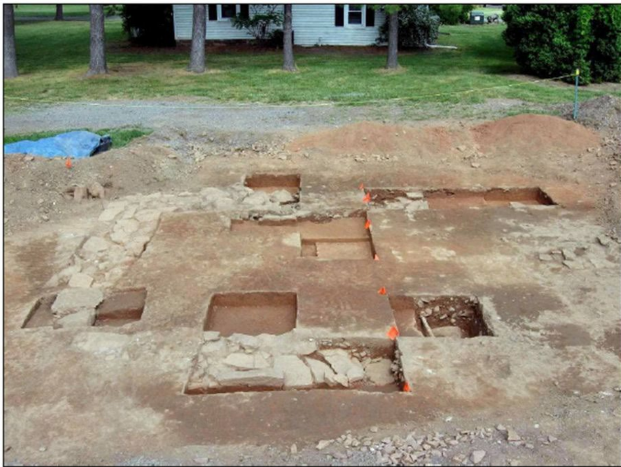
Figure 6-4. Overview of the Foundation (F-5), View to the East
