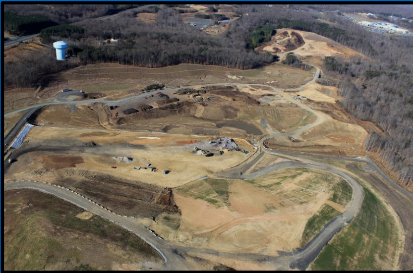
Prince William County Landfill
