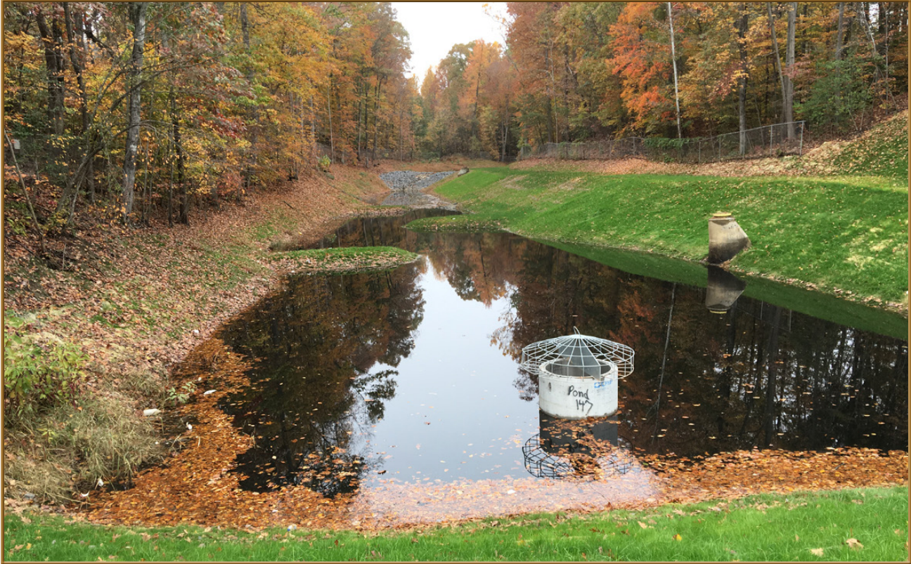
Powells Creek Watershed Water Quality Retrofit
