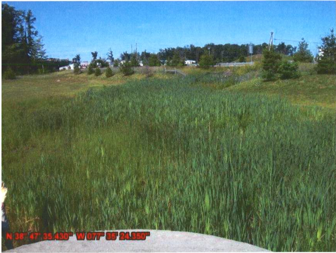
Photo 1: Large dry basin supporting wetland vegetation over about 33% of the basin
