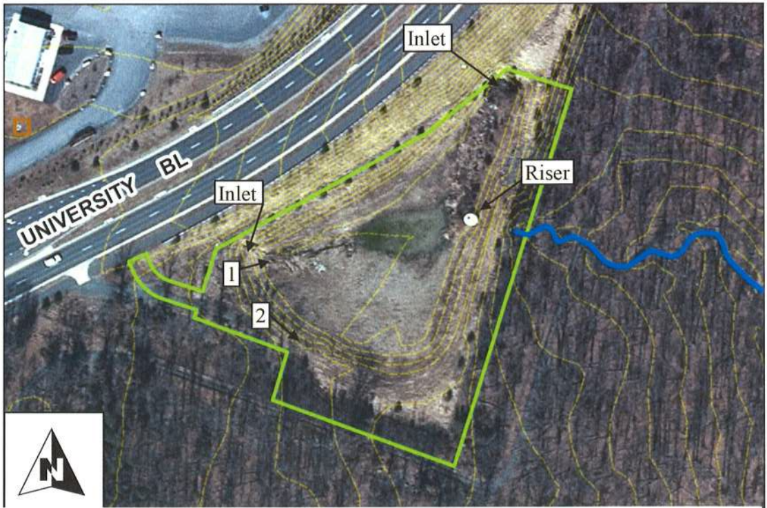
Existing Condition: Dry basin showing wet conditions and sediment load
