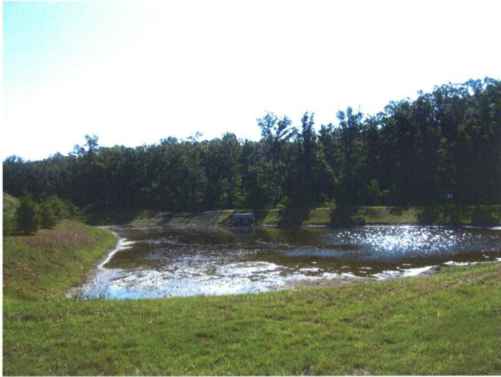
Photo 1: Site appears to be designed as wet pond, no forebays, and heavy sediment load
