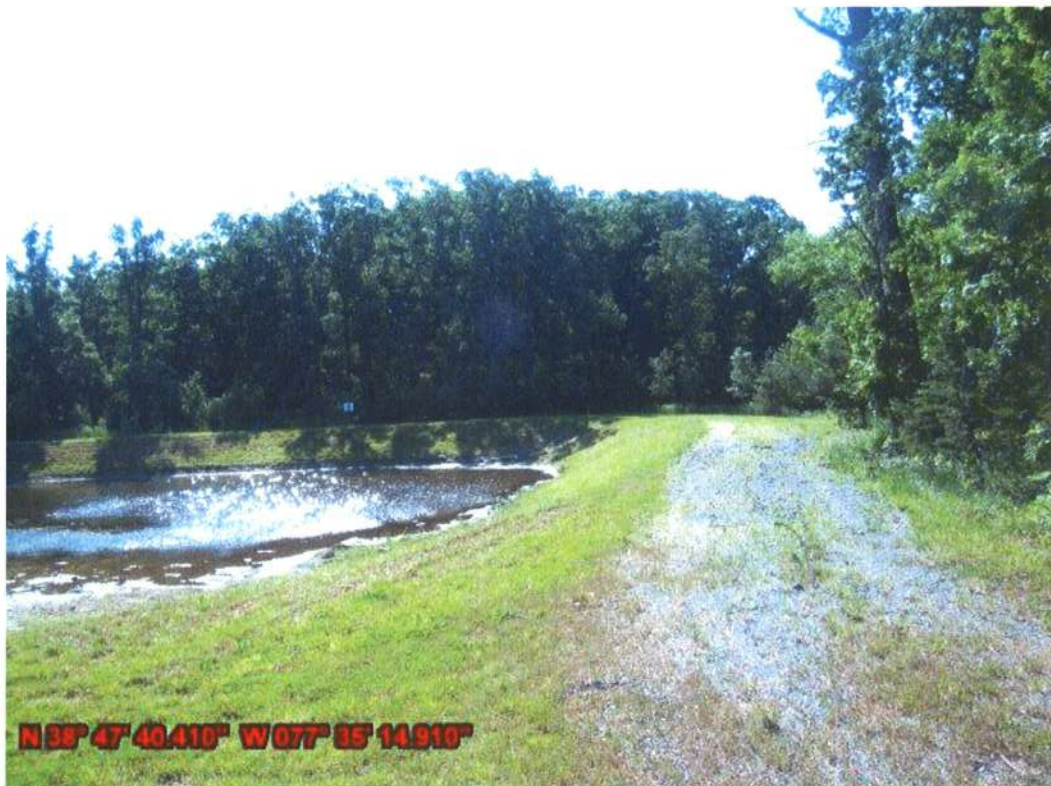
Photo 2: Service road provides easy site access for sediment removal
