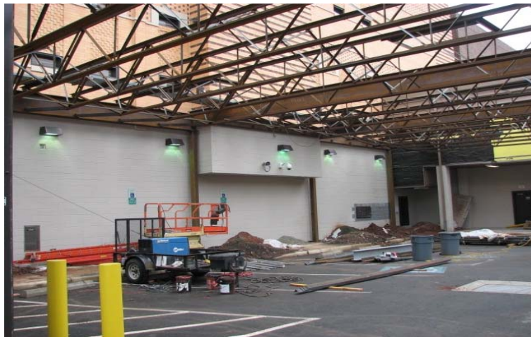
Construction of the Vehicular Sally Port
