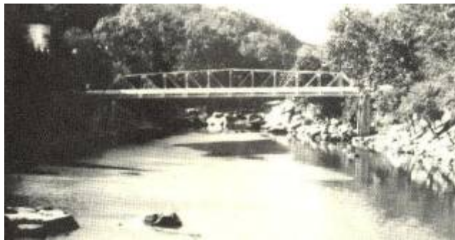
Steel Truss Bridge Over the Occoquan
