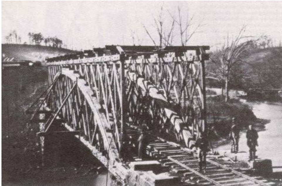
Orange and Alexandria Railroad bridge over Bull Run during the Civil War
