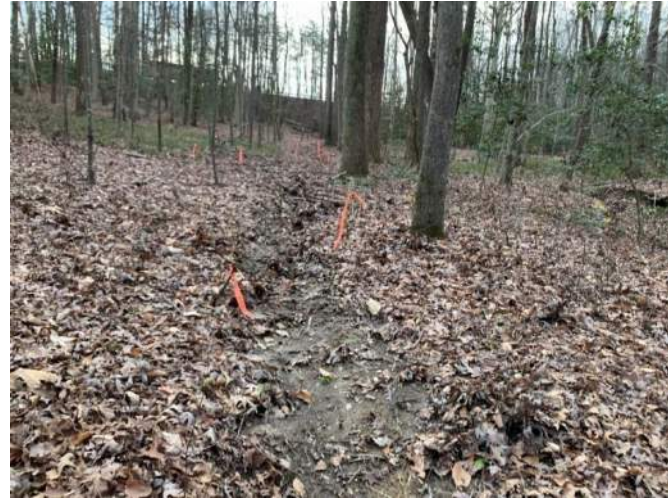
Photo #86: Representative Photo of system Z (EPH) looking upstream. Date: December 9, 2020
