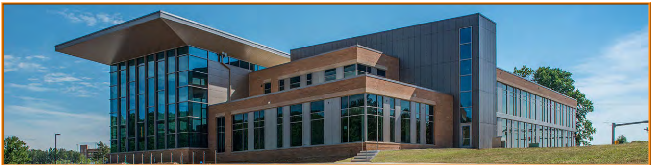
Northern Virginia Community College - Workforce Development Center
