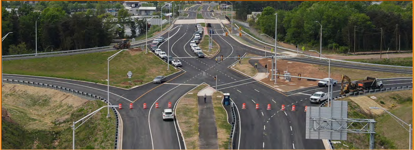
Balls Ford Road Interchange
