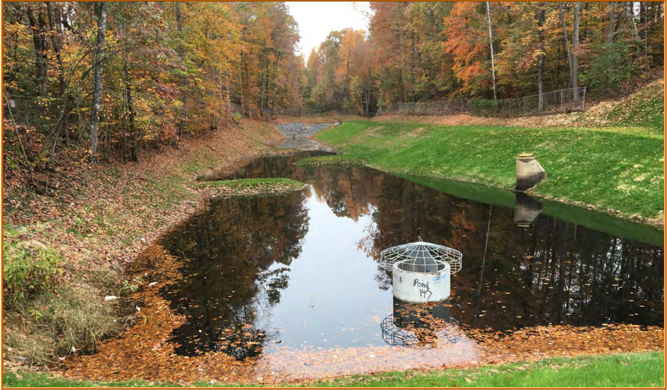
Powells Creek Watershed Water Quality Retrofit
