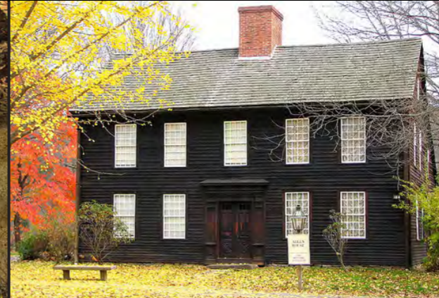
Old Deerfield Village Historic District, Franklin County, MA Corey P. Nasman
